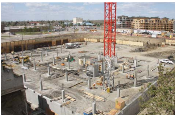
Community Centre construction as of May 14, 2008
